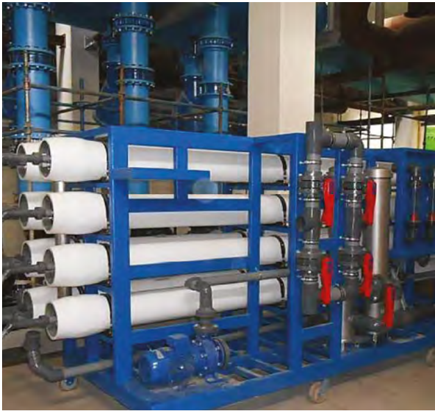
Reverse Osmosis Plant (for potable water)
