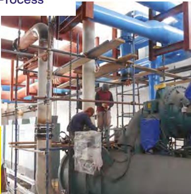
Electric Chillers Hook-up Process
