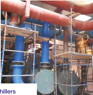
Electric Chillers Hook-up Process
