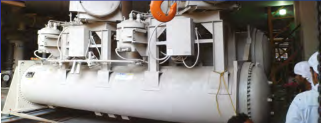
Mounting the DAIKIN Electric Chillers
