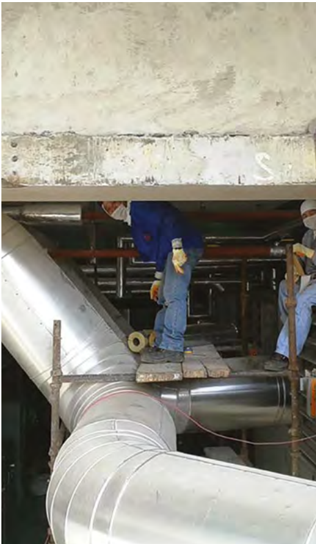
Exhaust Pipe Ducting + Cladding
