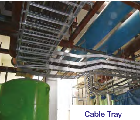
Cable Tray Arrangement
