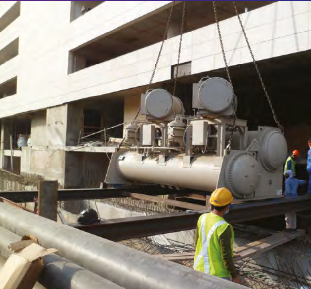
Unloading the DAIKIN Electric Chillers
