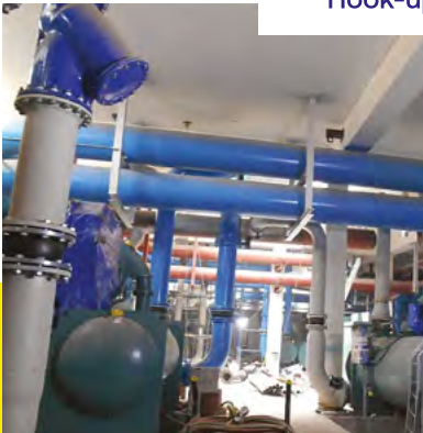
Electric Chillers Hook-up Process
