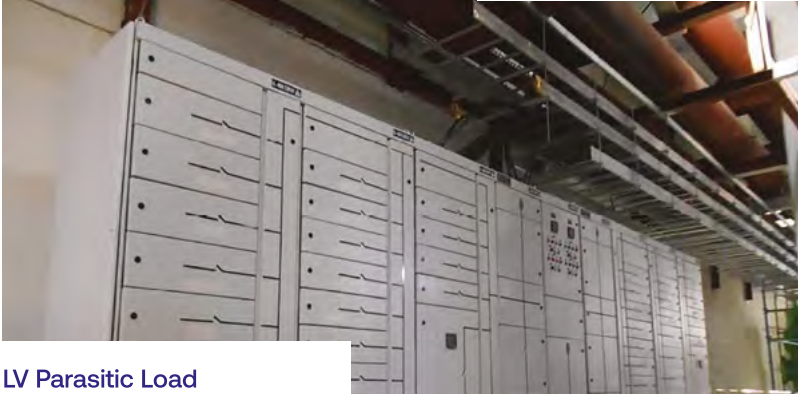
LV Parasitic Load (Designed & Manufactured in Al Aman Factories)
