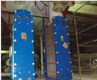
Hot Water Heat Exchangers
