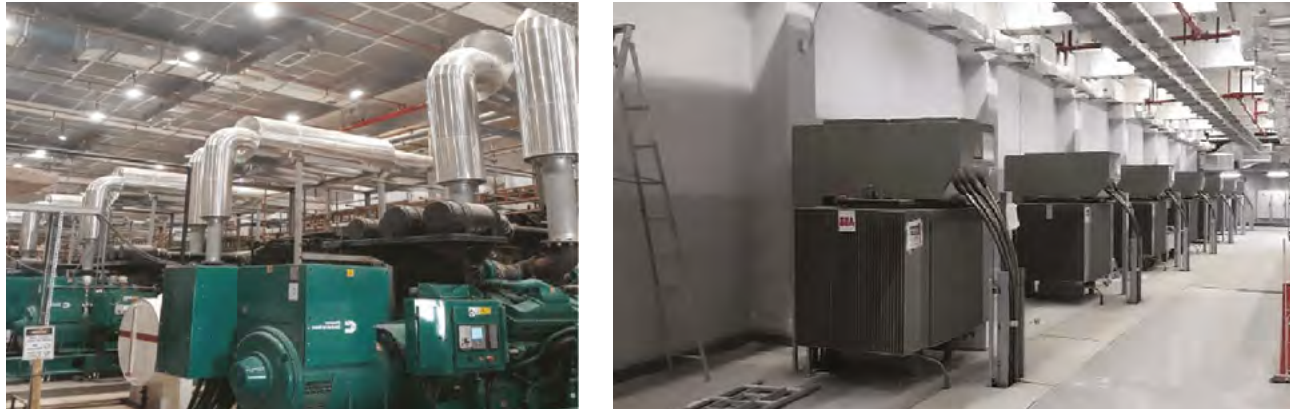
Scope of work done
