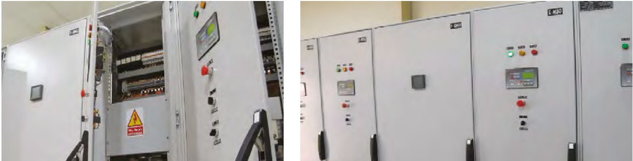
Scope of work done
