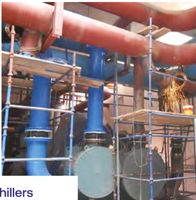
Electric Chillers Hook-up Process
