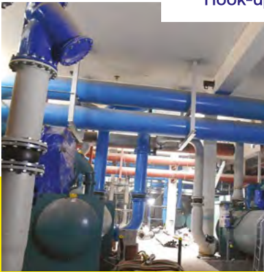
Electric Chillers Hook-up Process
