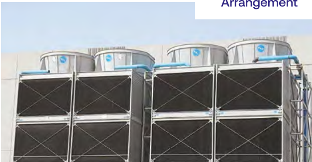
Cooling Tower Arrangement
