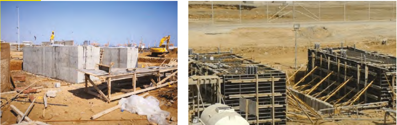
Scope of work done
