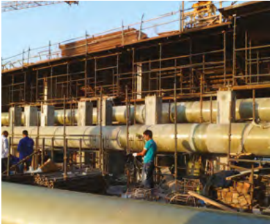
GRP Piping System for Water
