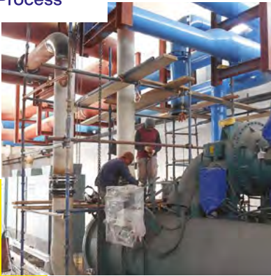
Electric Chillers Hook-up Process
