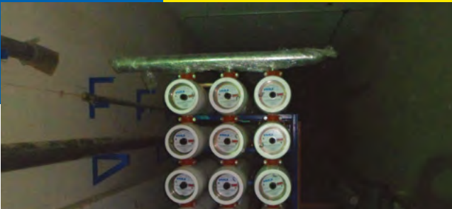
Reverse Osmosis Plant (for potable water)
