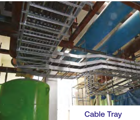
Cable Tray Arrangement
