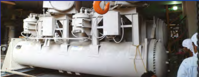
Mounting the DAIKIN Electric Chillers
