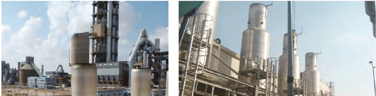
Scope of work done
