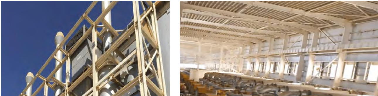
Scope of work done
